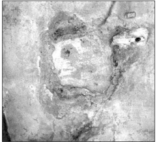
Illustration 24: Closed ventilation hole in the airlock of Crematorium I.
